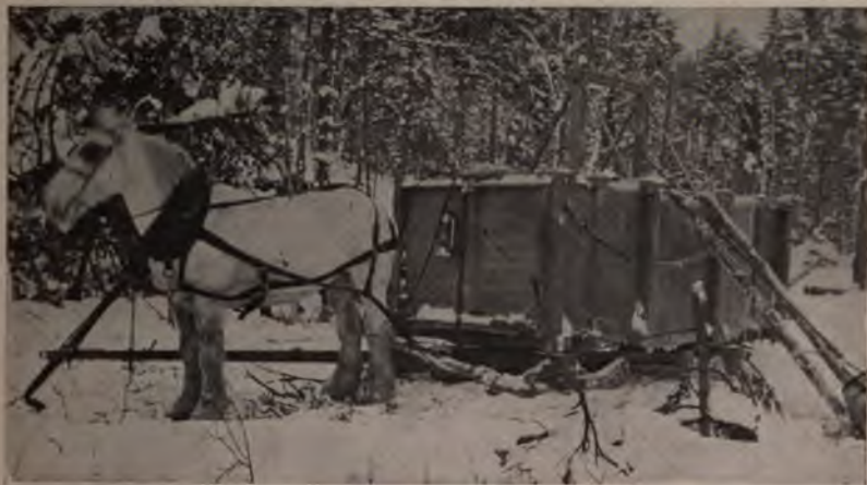
FIG. 41. — A Sprinkler being filled with Water from a Brook. Maine.
